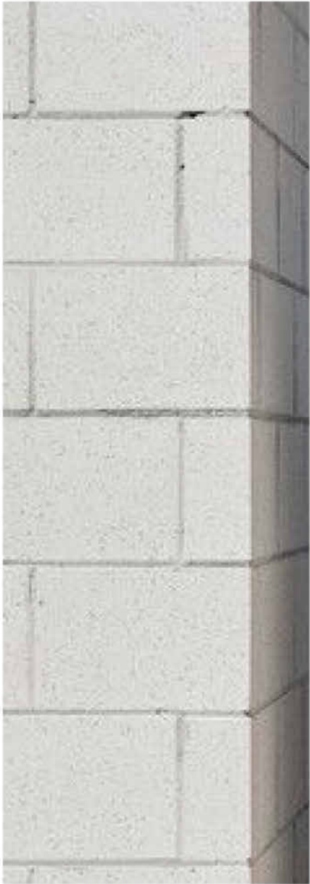
BL01 - CONCRETE BLOCK WALL
