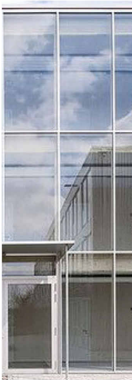
GL01-03 - FACADE GLAZING: VISION AND SPANDREL GLASS
