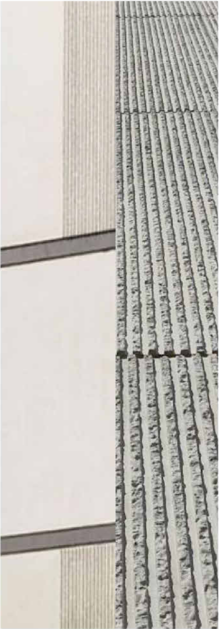
CON02 - SMOOTH AND TEXTURED PRECAST CONCRETE PANELS
