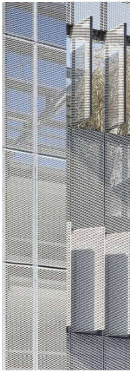
MT01 - PAINTED EXPANDED METAL MESH AND FINS
