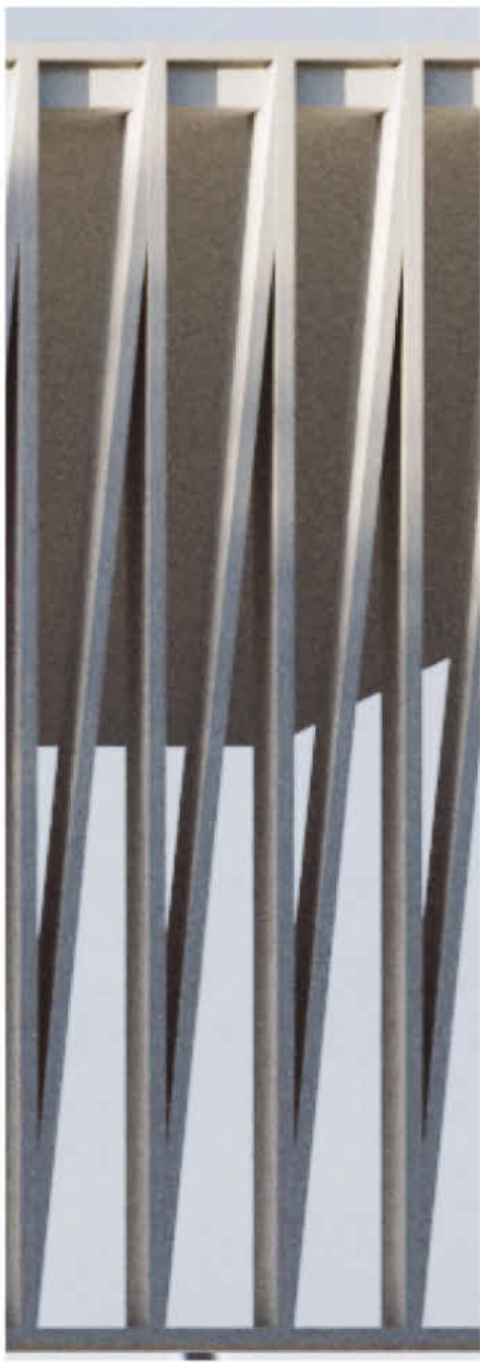
MT02 - PAINTED PROFILED STEEL SCREEN
